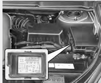
Engine compartment fuse panel
