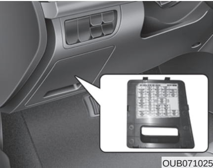
Instrument panel fuse panel
