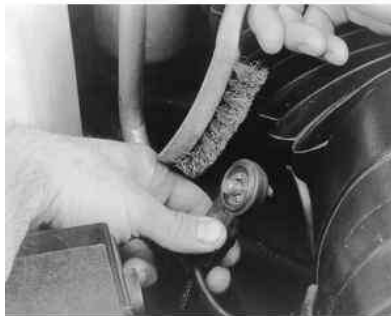
Fig. 3: A wire brush may be used to clean any corrosion or foreign material from the cable
